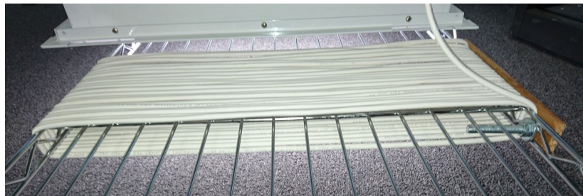
Figure 16. Example side view of bent cable.
