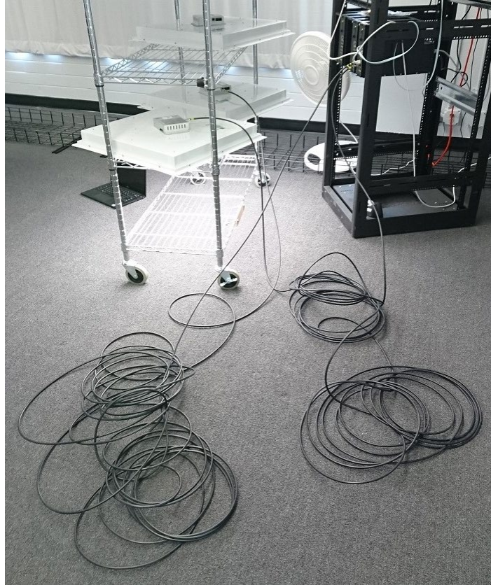
Figure 15. Example of cable prior to bending.
